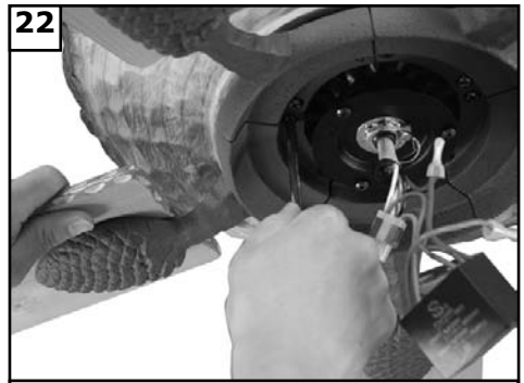
22 Check the motor for plastic shipping stabilizer tabs, and remove them if they are present. Attach blade assembly to motor using the motor screws and washers provided. Tighten screws securely.
